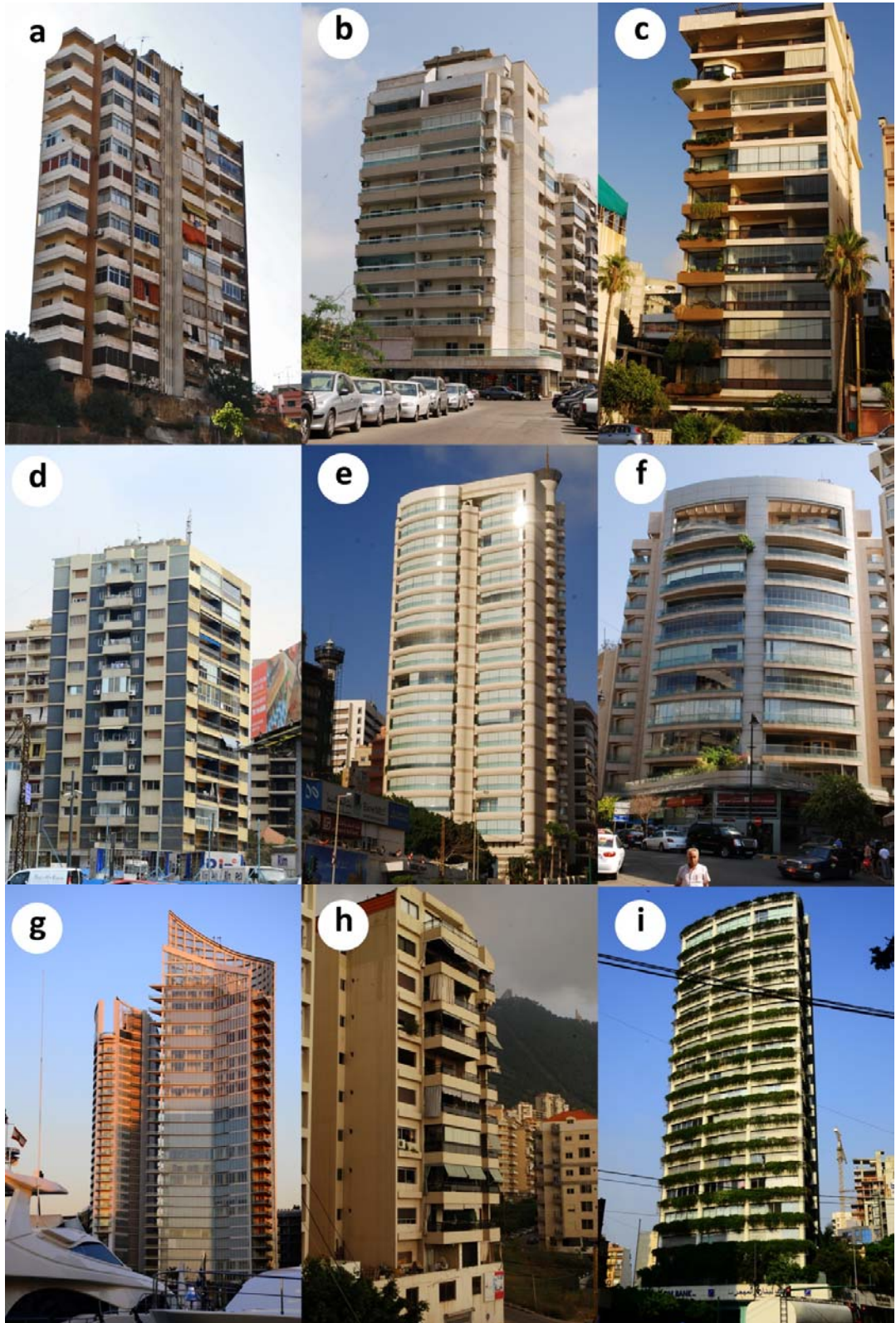
Figure 2.14 A selection of medium height residential buildings with the balconies always present, some of which have been glazed to gain extra space, while others have only external awnings. Also, some façades are not stone clad (a; c; d & h). Example (g) from downtown Beirut is an atypical all-glass residential building.
