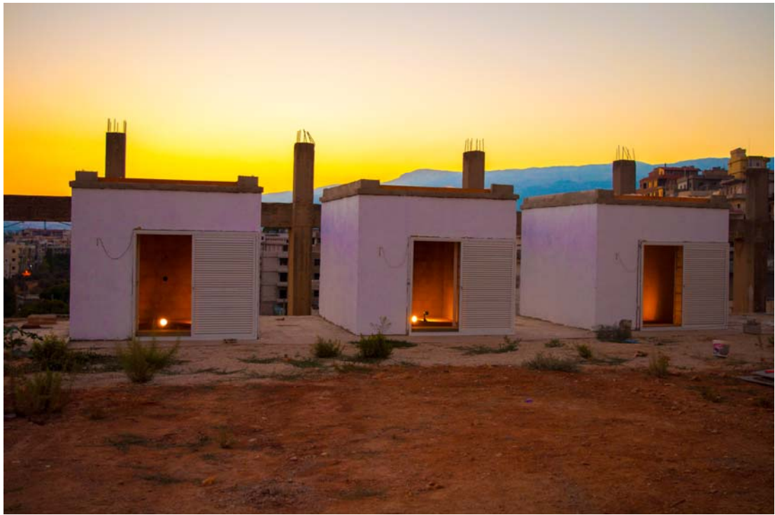
Figure 6.1 The three completed test cells showing the internal lights on, just before sun rises from behind the mountains.
