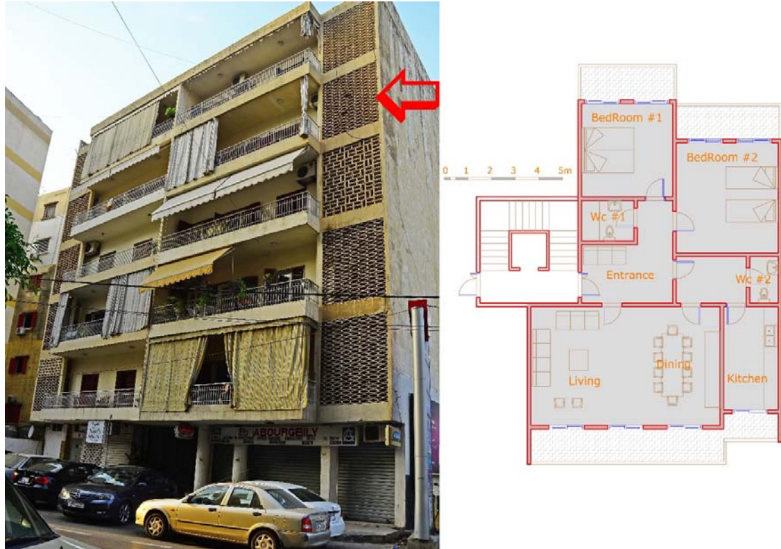
Figure A1.2 The building and the corresponding plan of half the floor.
