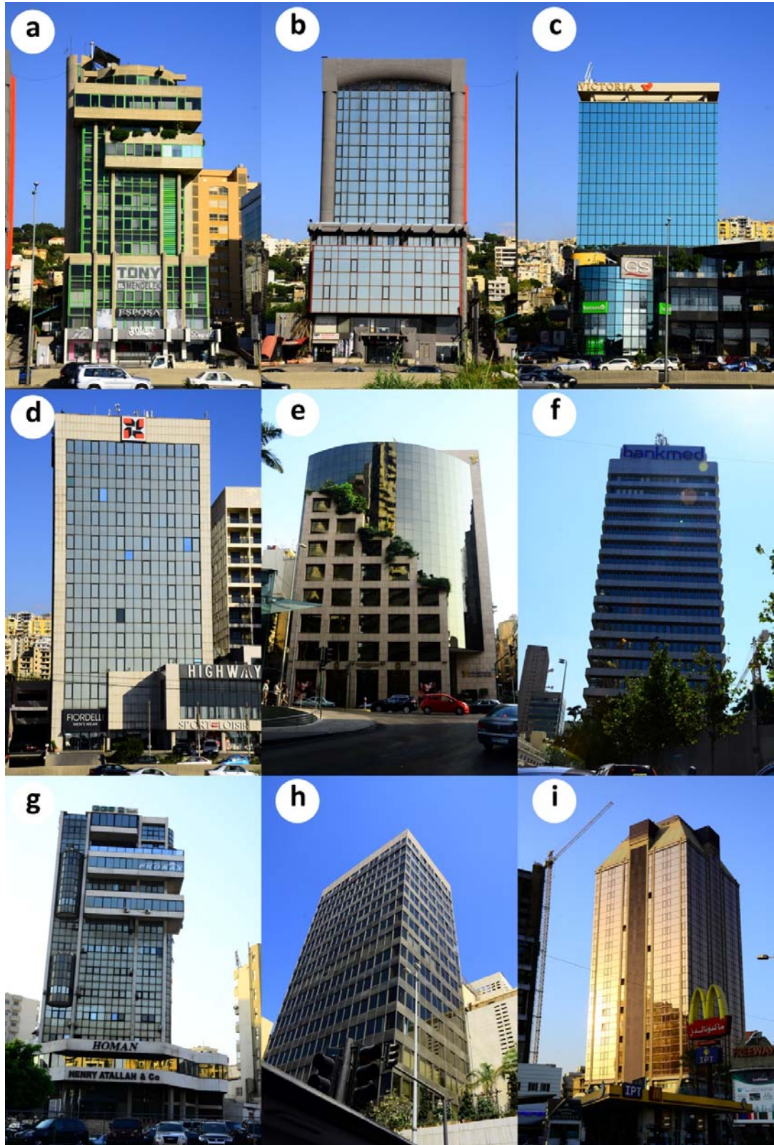
Figure 2.15 Selection of office buildings showing the typical typology: no balconies, with either full glazed façade or alternating glass and opaque strips.
