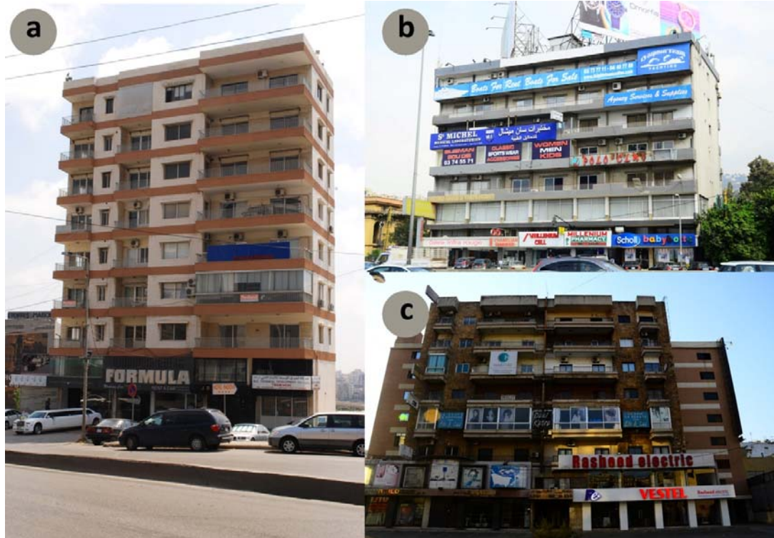
Figure 2.16 Typical mixed use or shifted function from residential to office: balconies are present, some of which have been glazed to enlarge the internal space. Advertisements are clearly exposed to promote the business.
