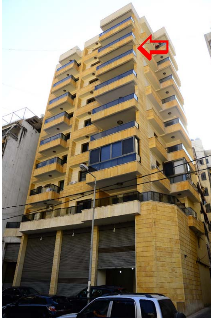
Figure 0.6 Front (east) main façade with the North side façade. The monitored apartment is on the 7 th floor.
