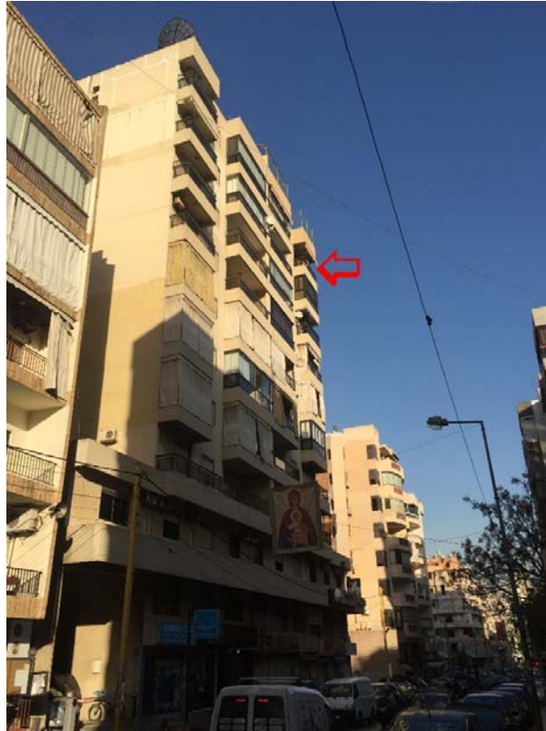
Figure 0.4 Back (north) facade of the Ghanimeh Building; the monitored apartment is on the last floor (left).
